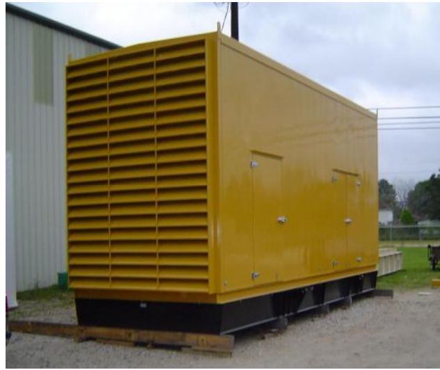
Plate 8.2. Generator sound attenuation house
