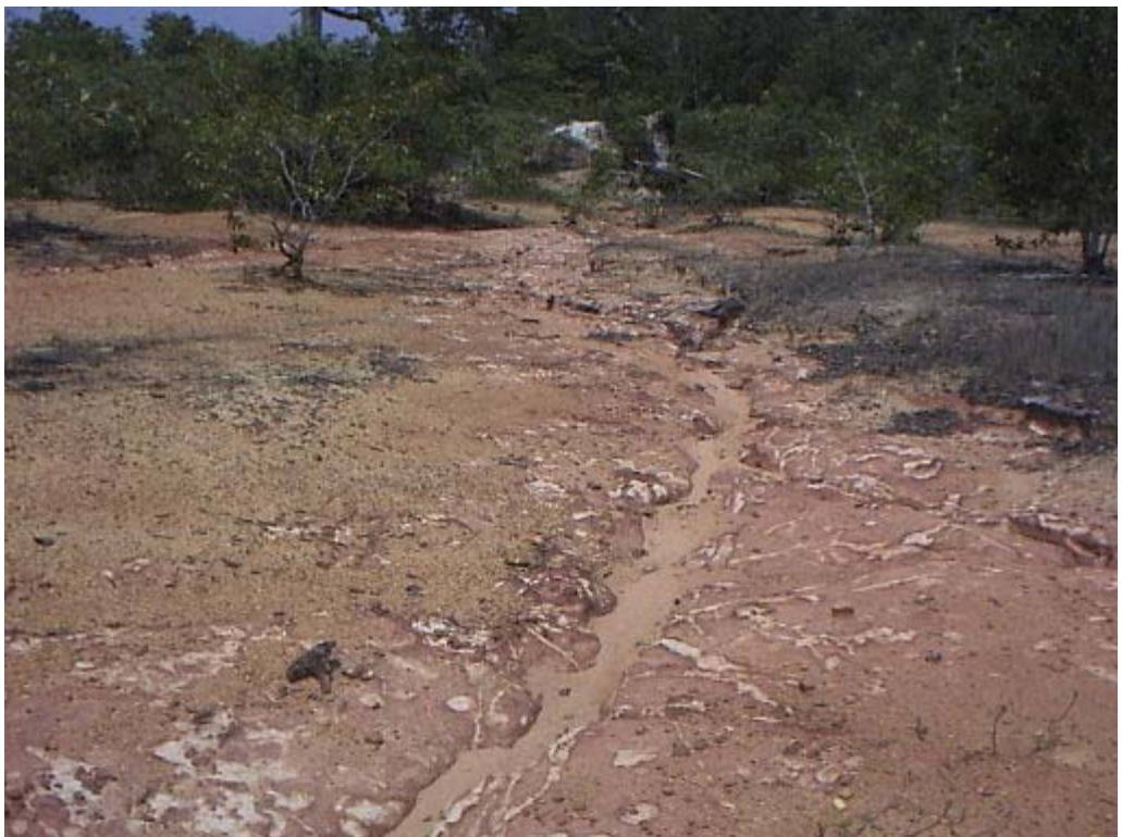
Plate 2: Typical erosion channel running along slope of ridge. Frame shows effect of erosion on exposed ground. These channels are along the southern slope.
